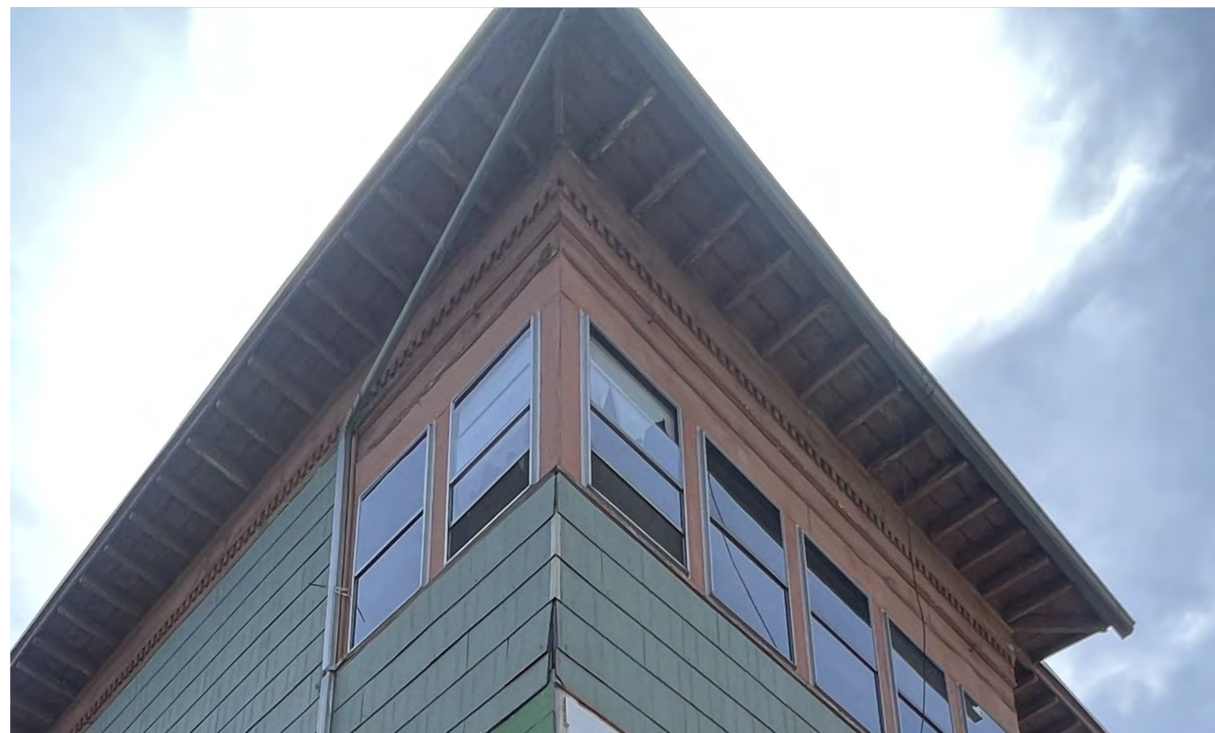
EXISTING ROOF DENTAL SCALE: NOT TO SCALE
